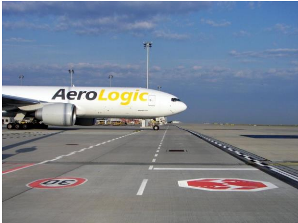
here: apron 4, northern operation street (taxi street)
